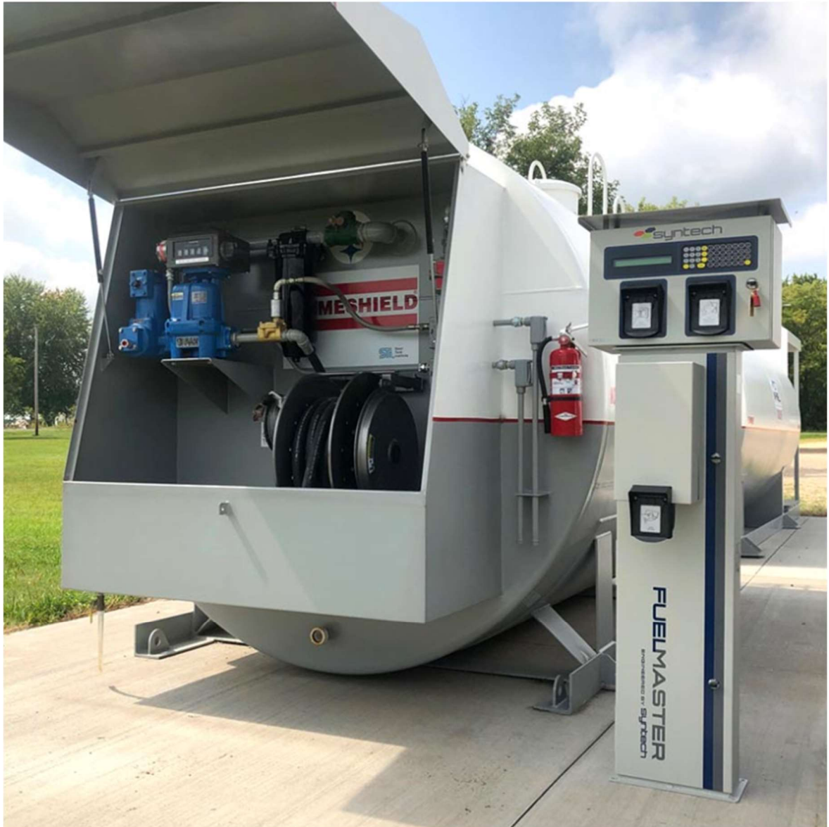
Image 11: View of TYPICAL Packaged refueling system
