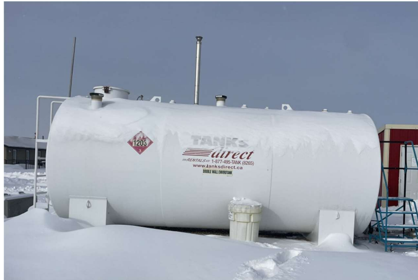
Image 1: View of AVGAS tank and spill kit
